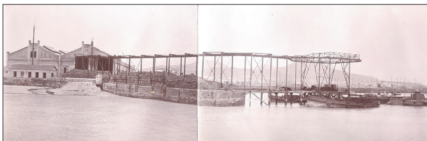
Miller's electric coal conveyor.
