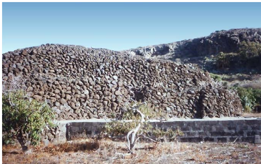
Fig. 16 - Another Grancanarian one-step "pyramide" from Los Pasos de Herrera, Valle de los Nueve, Telde (photo: FEDAC/Carta Etnográfica de Gran Canaria). Type C with a relatively high first step. One can realize unusual notches in the supporting wall, similar to fig. 7. In the foreground a modern wall.
