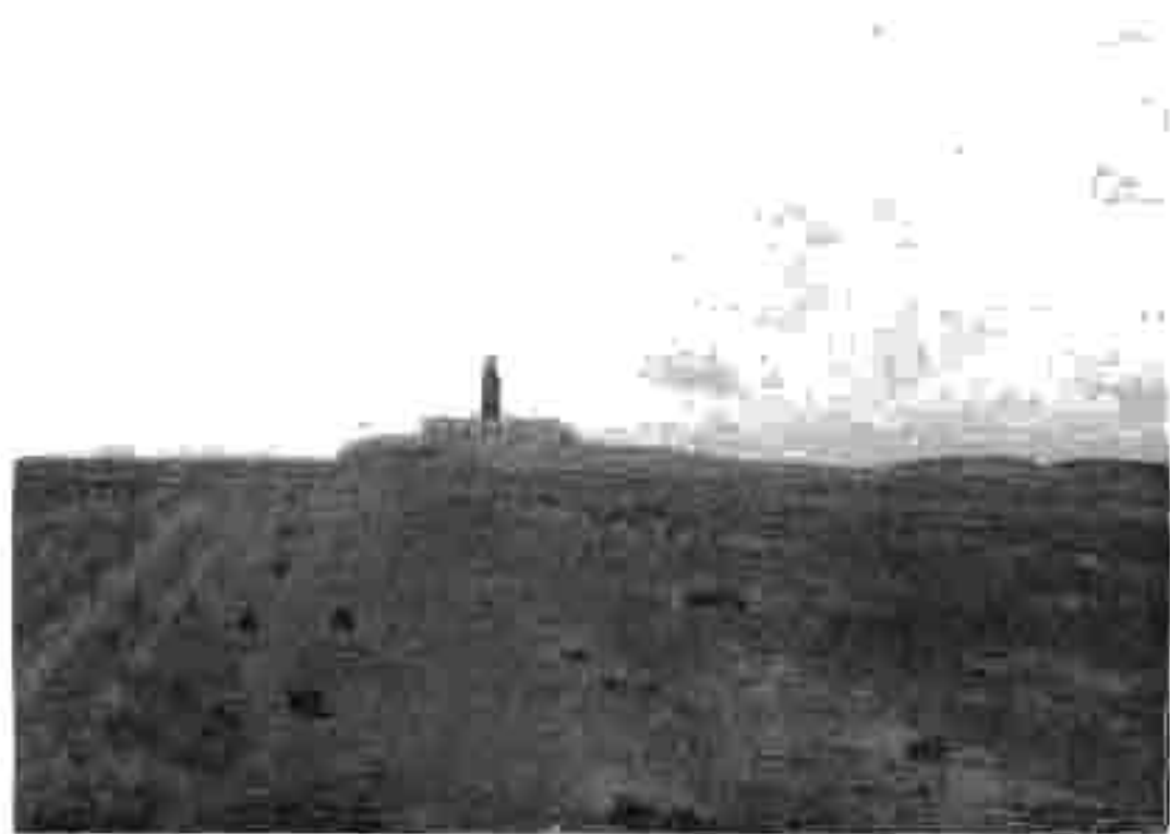
View of the tower
