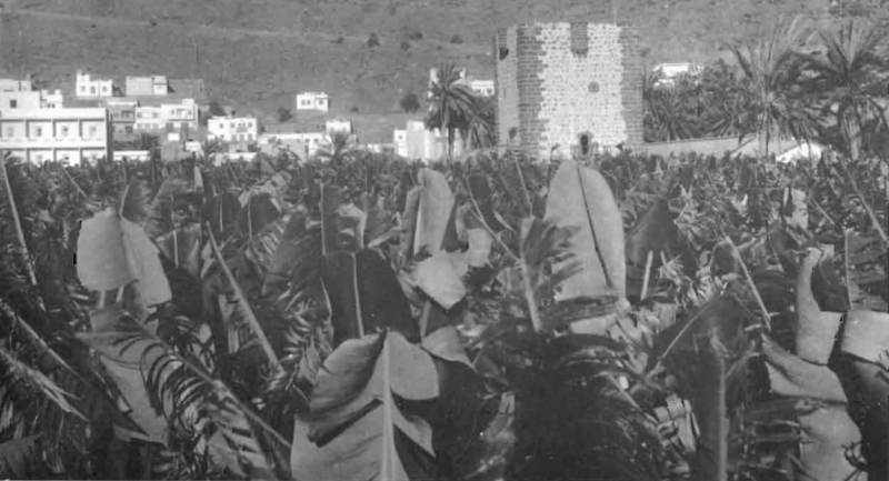
24. Gomera: the fifteenth century Torre del Conde, oldest building in the Canaries still intact and in use, rises above the banana plantation which now grows where the waves once lapped up against its walls (pp. 149-153)
