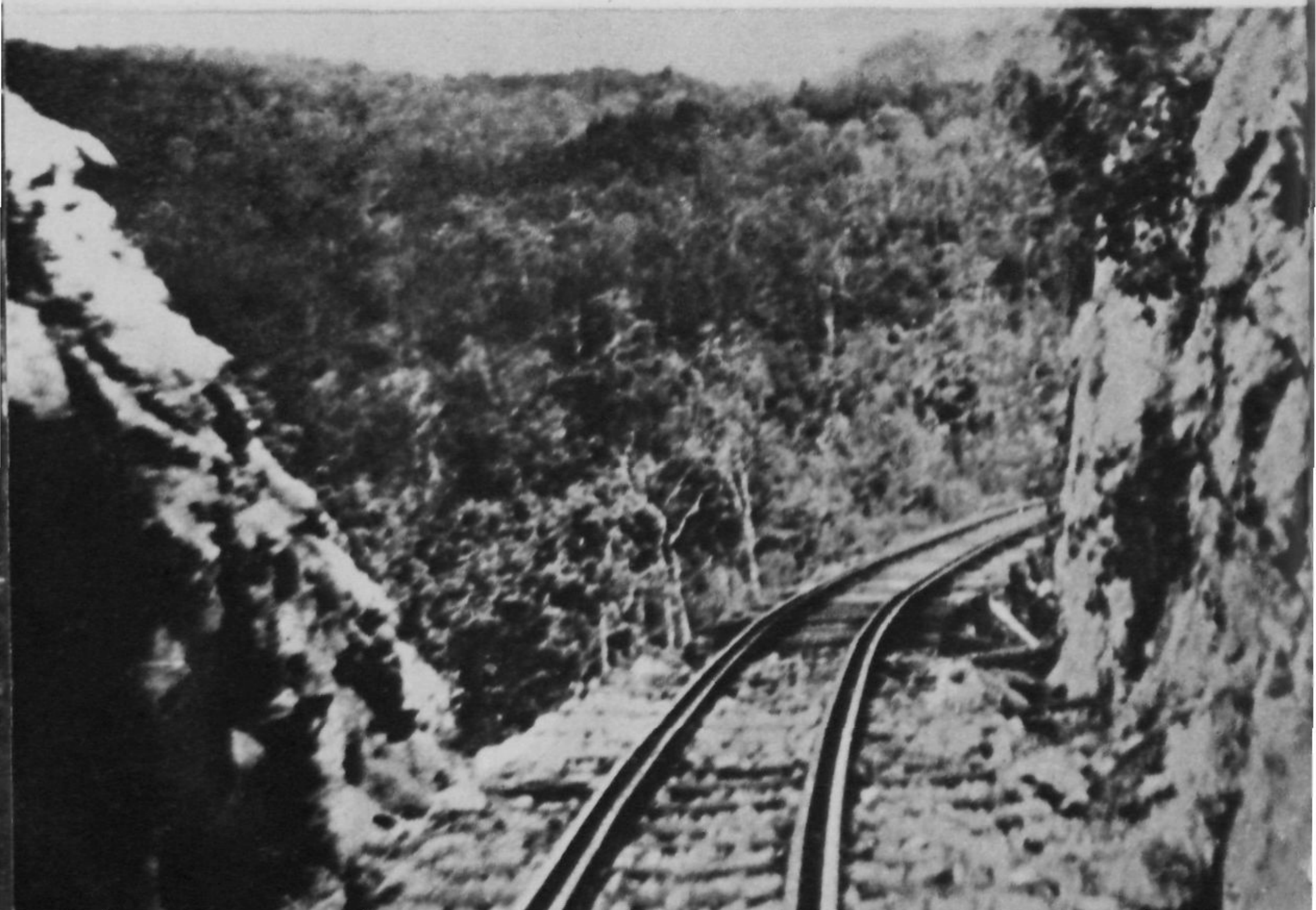
A section of the railway near Kinsayok cut through virgin rock
