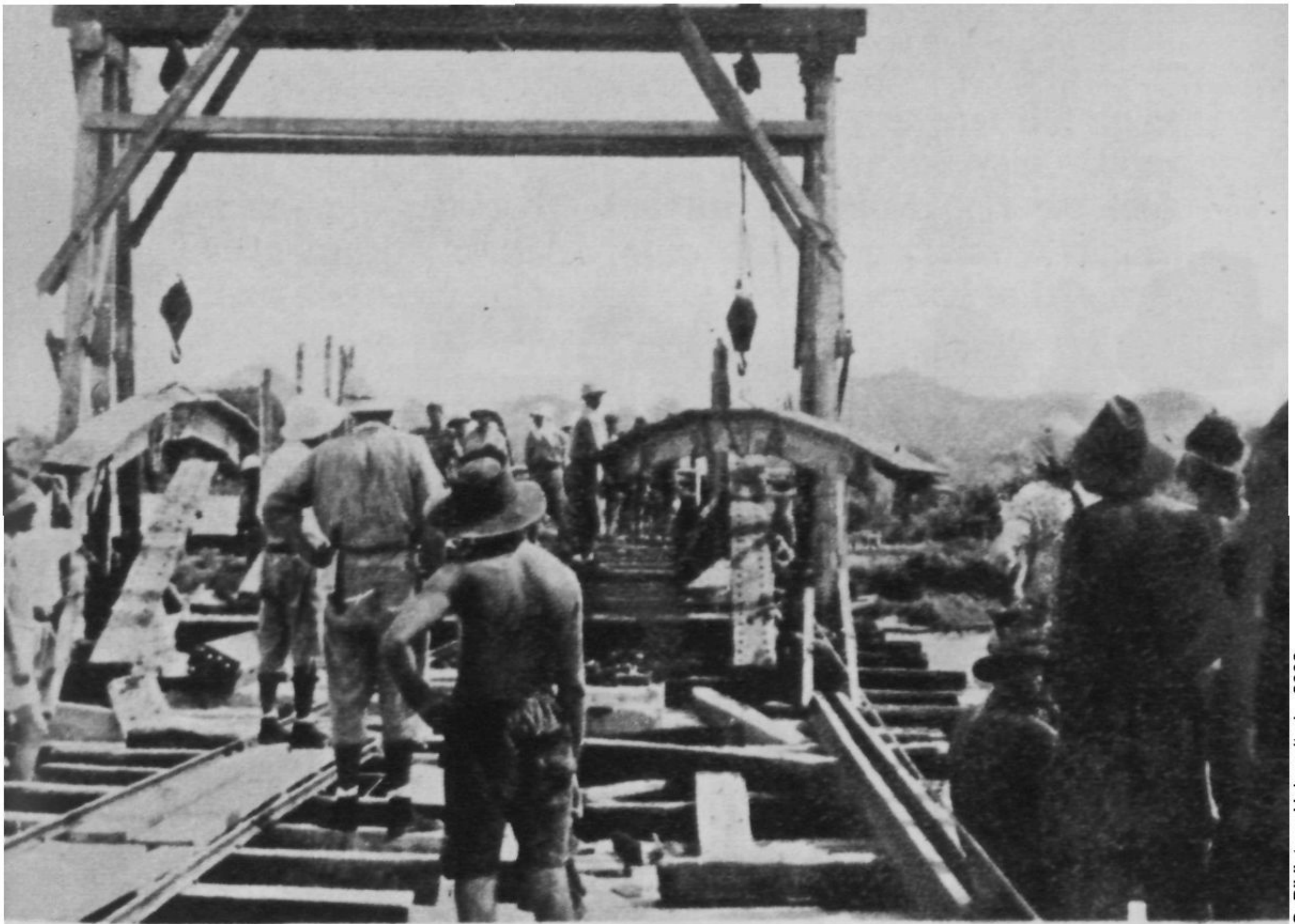
Building the bridge at Tamuang
