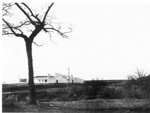
PARTIAL VIEW OF THE STUDIO-WORKSHOP IN SAN SEBASTIAN DE LOS REYES, Madrid Work of the Architecte Antonio Fernández Alba, 1960-63
