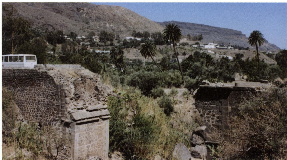
Photo 6. The Rosiana landslide has been reactivated at least four times in the past (1879, 1921, 1923 and 1956). Some palm trees were tilted, many houses were destroyed and the old bridge collapsed because of the movements.
