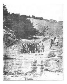
Figure 4. On the left branch a channel of 179 m length was built, with 32 steps, and variable width.
