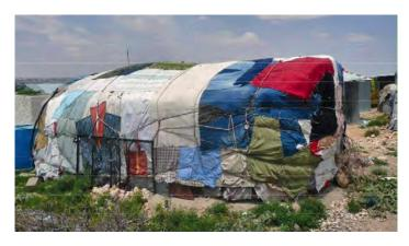
Figure 2. Buul Shelter (1991); self-constructed Shelter based on traditional Buul. Somalia.
