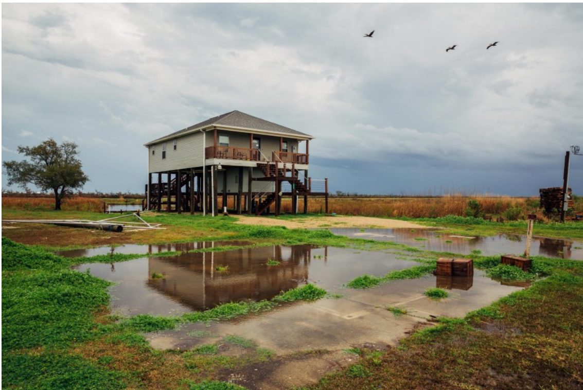
Fig. 11: Casa sobre pilares post-Katrina, Hopedale, LA 2015. Elevated post-Katrina house, Hopedale, LA, 2015.
