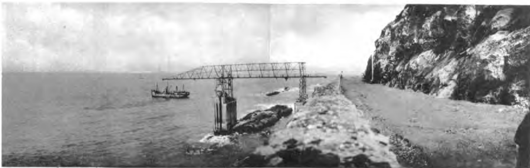
The Landing-place, Hermigua, Gomera. Note basket with passengers for the s.s. Taoro .
