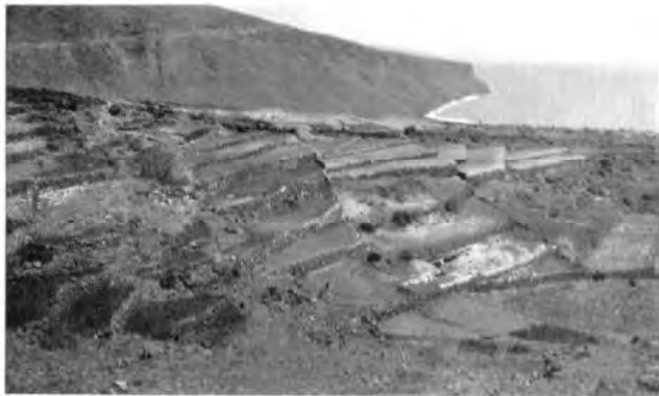
Remarkable Terracing on the Guimar-Fasnia Road.
