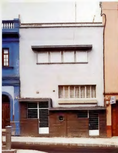
Casa O'Shanahan O'Shanahan House
