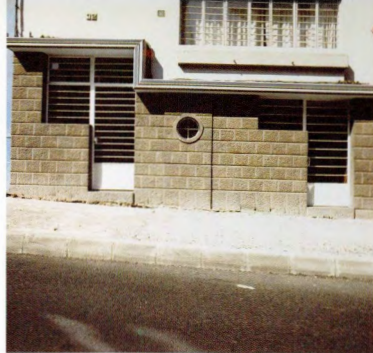
Casa O'Shanahan. O'Shanahan House
