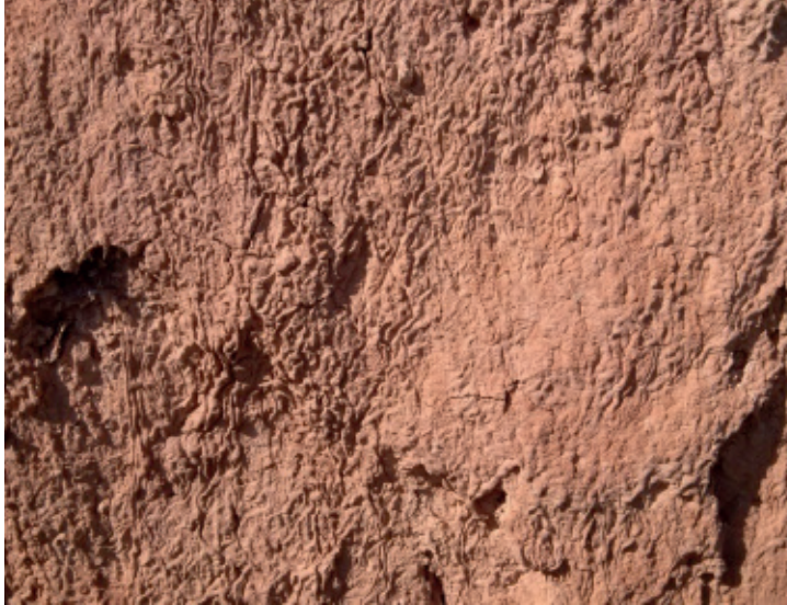
Figure 12: Clay and straw coated walls.
